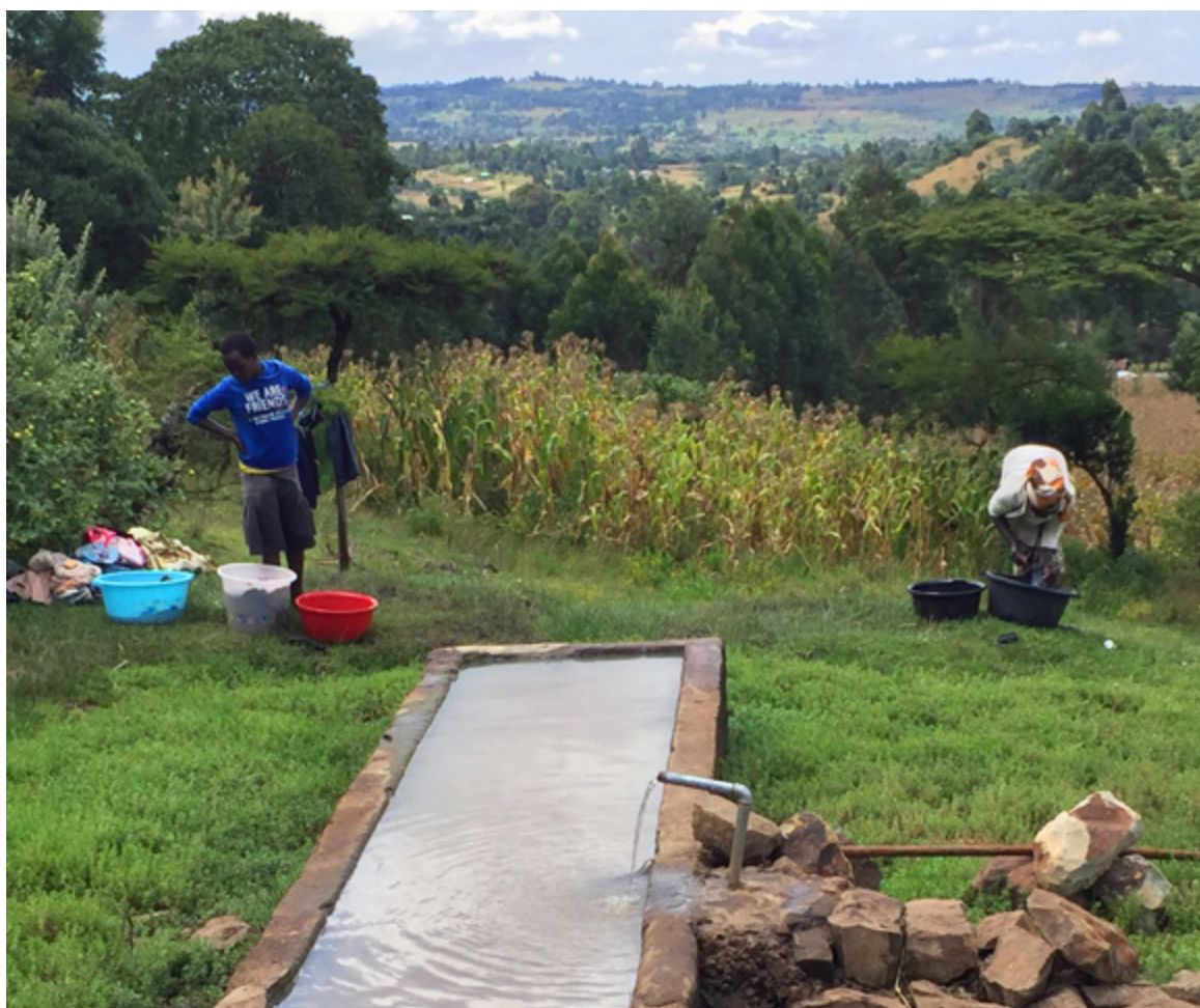
Water protection scheme which protects the source while providing safe, easy access to clean water (November 2019)
