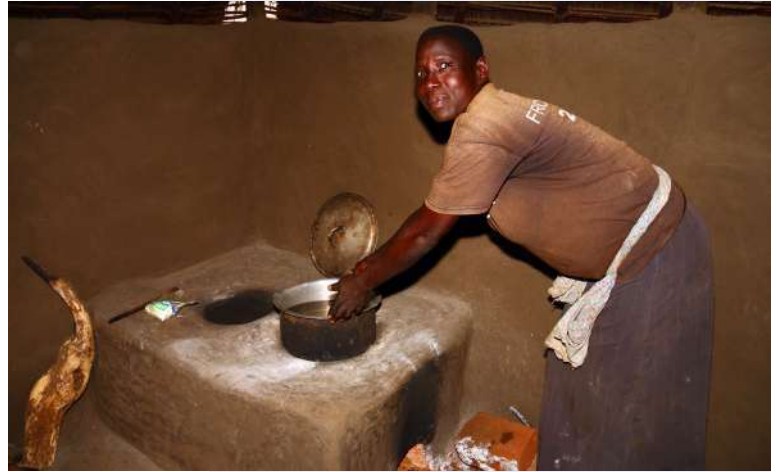
A smokeless stove installed in a local home in Uganda
