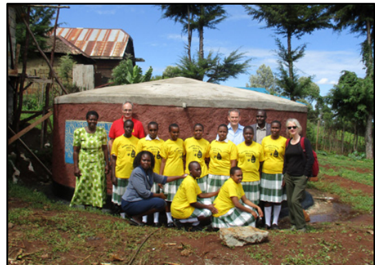
Chepseon Secondary School ferrous cement water tank
