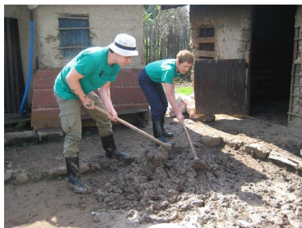
Eoin & Pauline getting to grips with mixing clay, water, sawdust & sand for the new stove
