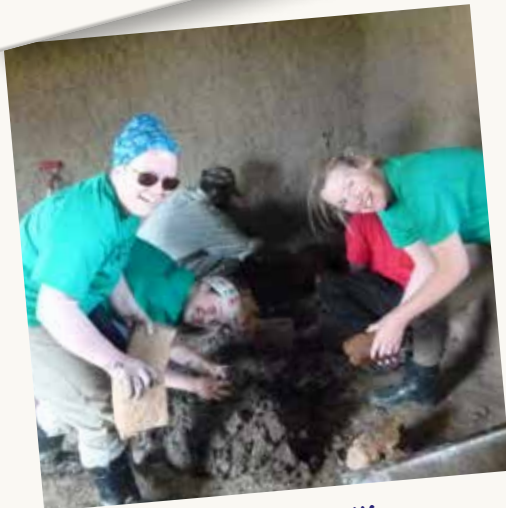
Volunteers installing smokeless stoves
