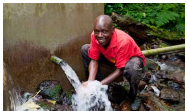
Reuben Koske, Field Officer at the intake of the gravity water scheme in Ndubusat, Kenya which provides water to 11,000 households
